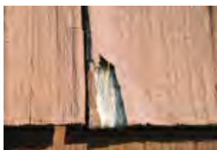
Not back primed. Primed over weathered wood .
